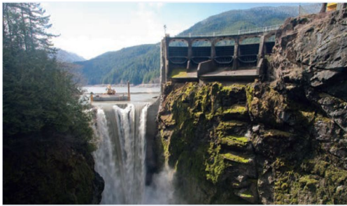
Source 6.51 The 64-metre-high Glines Canyon dam partially removed in March 2012
